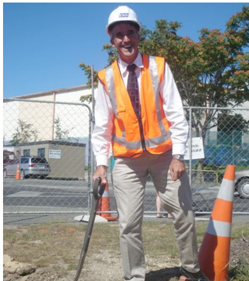
Mayor Richard Kempthorne gets work started on Richmond's new town centre.
