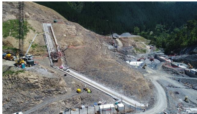
LHS plinth progress looking downstream, Dec 2020
