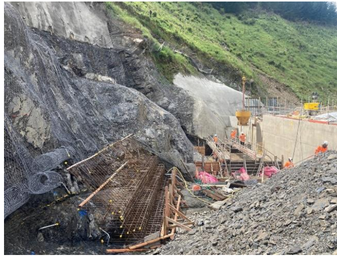
RHS plinth void buttress support concrete pour, Nov 2020
