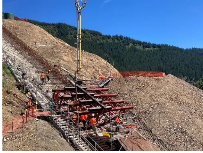
Pouring concrete in steep LH plinth section, Dec 2020
