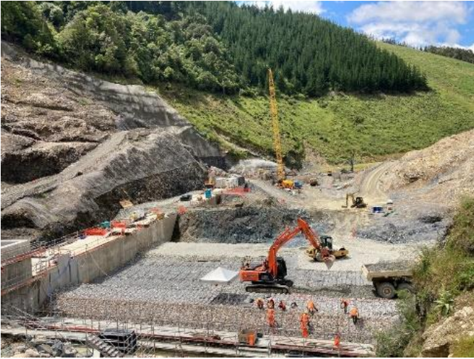
Overview of reinforced rockfill placement, Dec 2020
