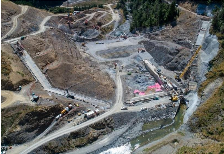
Aerial view of the site progress, February 2021
