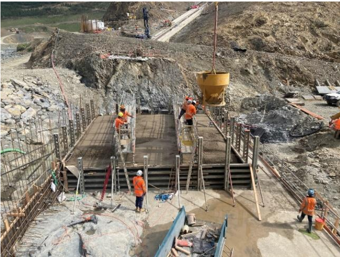
Pouring concrete in starter dam, Nov 2020
