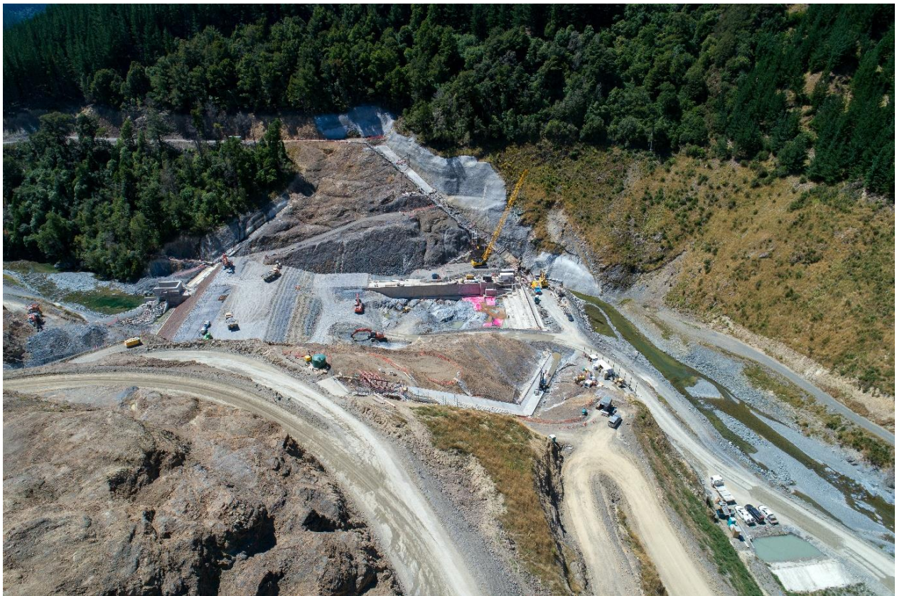
Construction Site, February 2021
