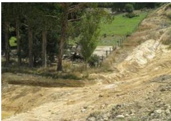
Figure 6-9 Sediment Control Diversion and Sediment Retention Pond
