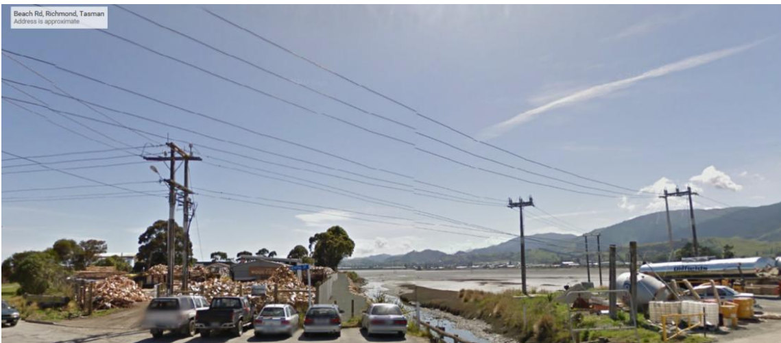
Google maps Beach Road, Richmond, 66KV lines
