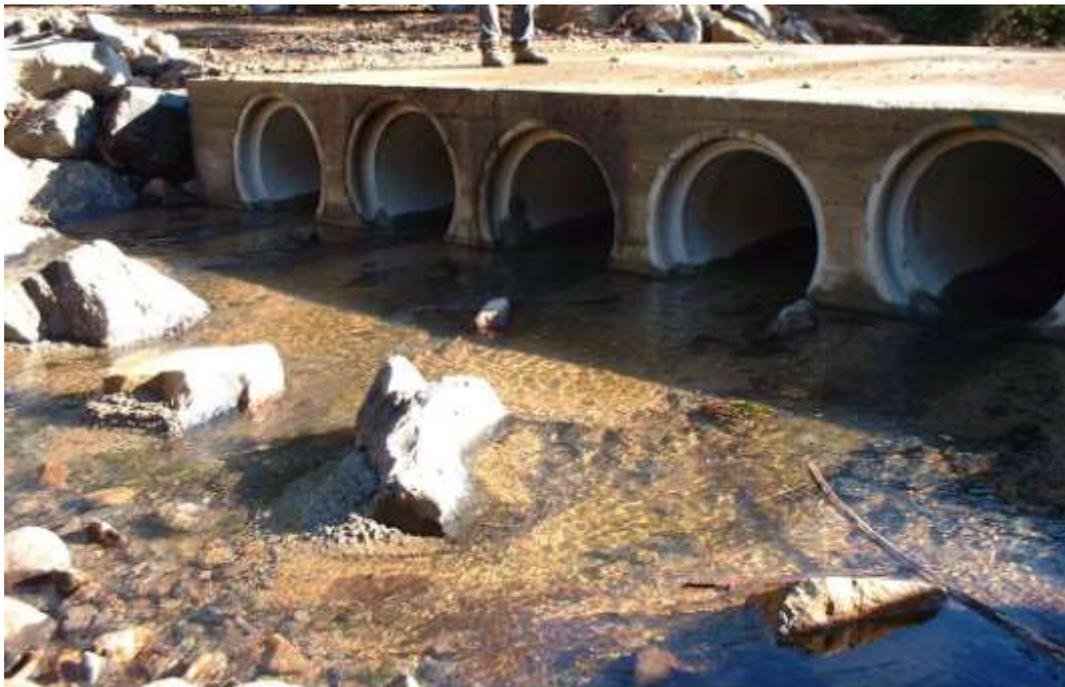
**Figure 7 Multi-barrel circular culvert with culvert pipes at different levels to cater for high flows and low flows**
