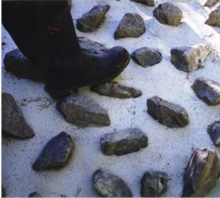
**Figure 10** Rocks can be cemented into the base of waterway crossings and/or to the aprons of culverts to ensure that there are areas of low water velocity available to aid fish passage and sediment which is appropriate for invertebrates is retained within the structure
