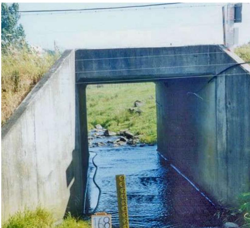
**Figure 8 Single box culvert**
