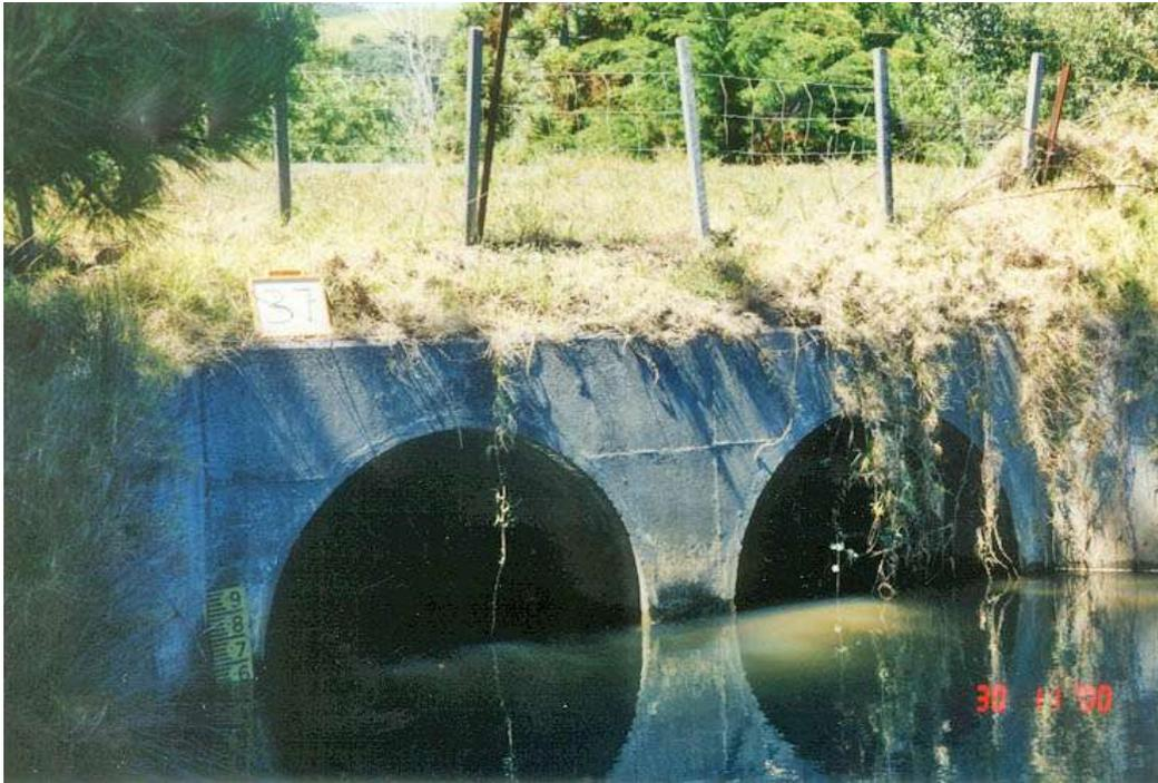
**Figure 6 Typical multi-barrel circular culvert**
