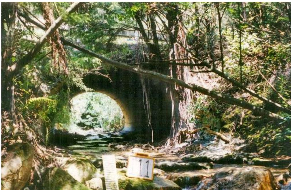
**Figure 2 Single barrel arch culvert**
