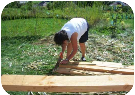
We cut the bamboo poles to the right size.
