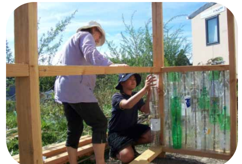
We slotted the poles into the frame.
