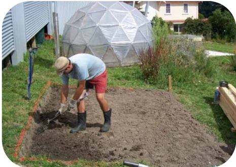
Aaryn Barlow, Master Builder, dug the foundations.
