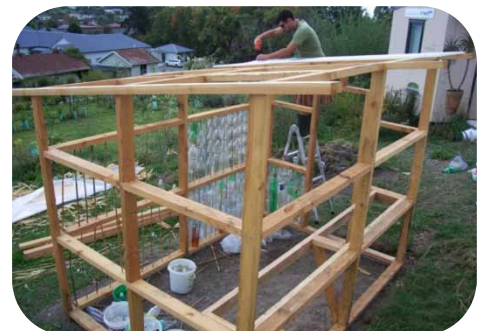
Aaryn put the roof on.
